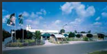
Silikal production and administration in Mainhausen, near Frankfurt/Main, Germany.
