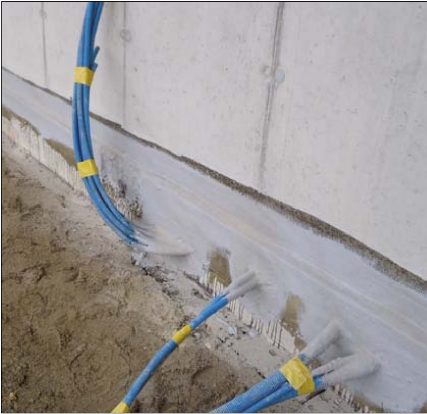
Joint seal with cable lead-throughs
