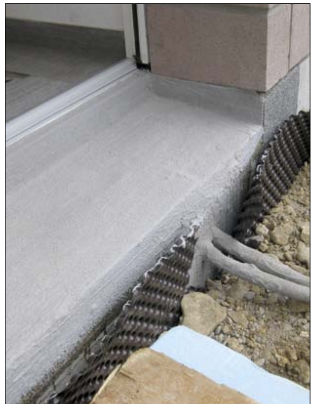
Threshold sealing
