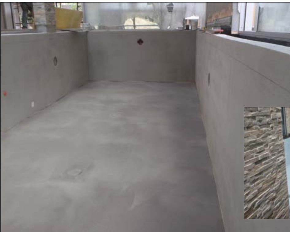
Swimming pool seal with subsequent tiling
