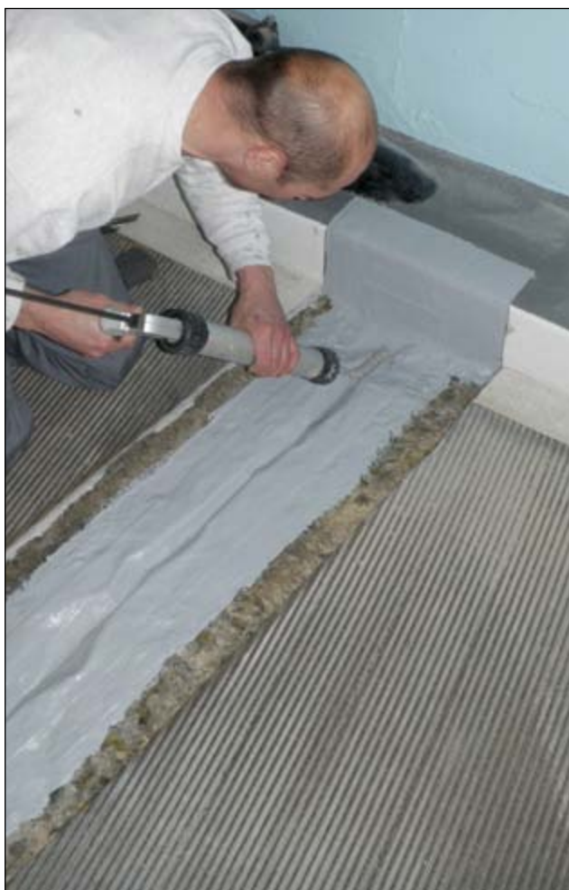
Movement joint/dilatation joint
