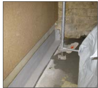
Change of material/joint seal
